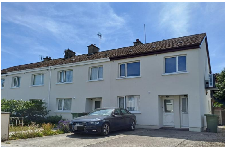
Energy Retrofit works completed at Seamount Drive Kilcoole 2025.
